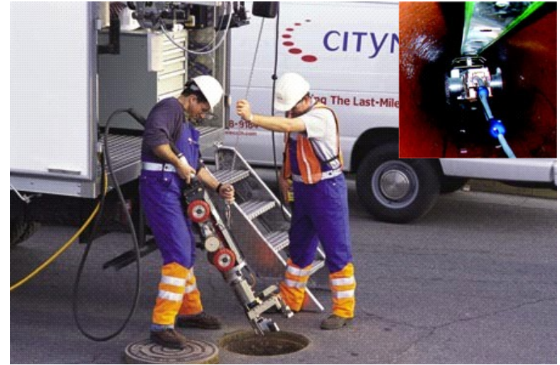
Figure: Fiber cables in sewage systems (source: CityNet, CableRunner)
