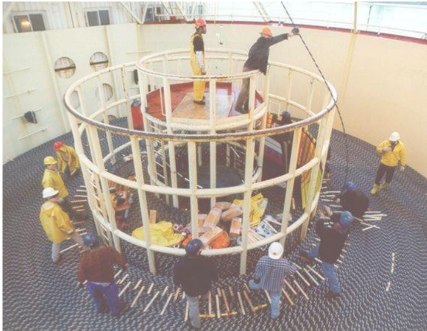
Figure: Feeding of cable onto ship storage (Canada, 2000)
