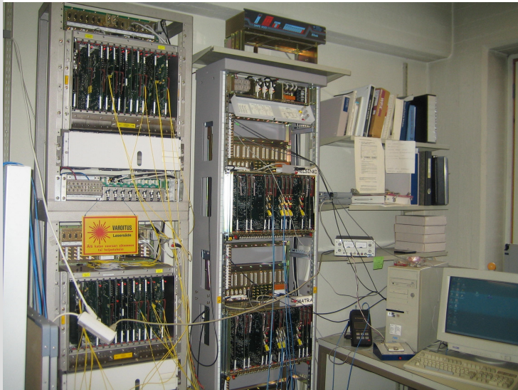
Two STM-16 and three STM-1/4 DCS in Comlab, TTK
