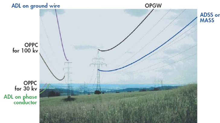
Figure: Fiber cables deployed on power transmission lines (source: Alcatel)
